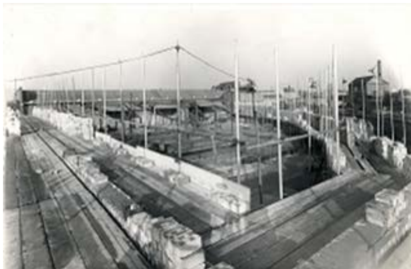
Veneer shop extension, 1954
