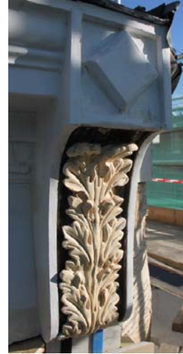
Restored corbel above shopfront.
