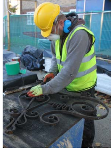
Restoring wrought iron sign bracket.
