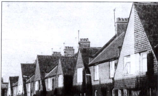
● Westmoreland slates hung on gable ends in a rhythm are an important local characteristic
