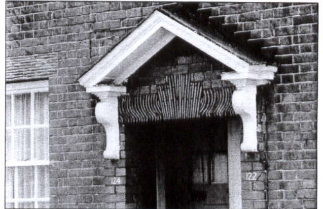
● Wavy tile details on edge lintels under classical corbels and pediment
