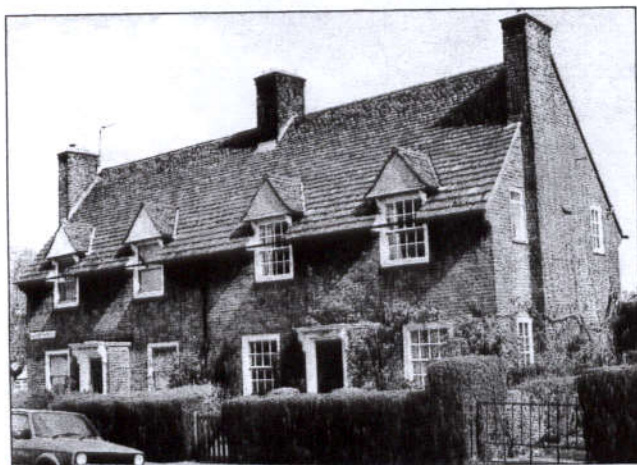
● The use of receding slates to emphasise perspective and give a traditional hand made feel to the roof
