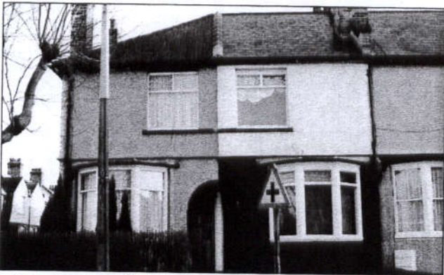
● The unfortunate effect of painted brick, replacement windows and doors and loss of hedge combine to remove the character of these houses
