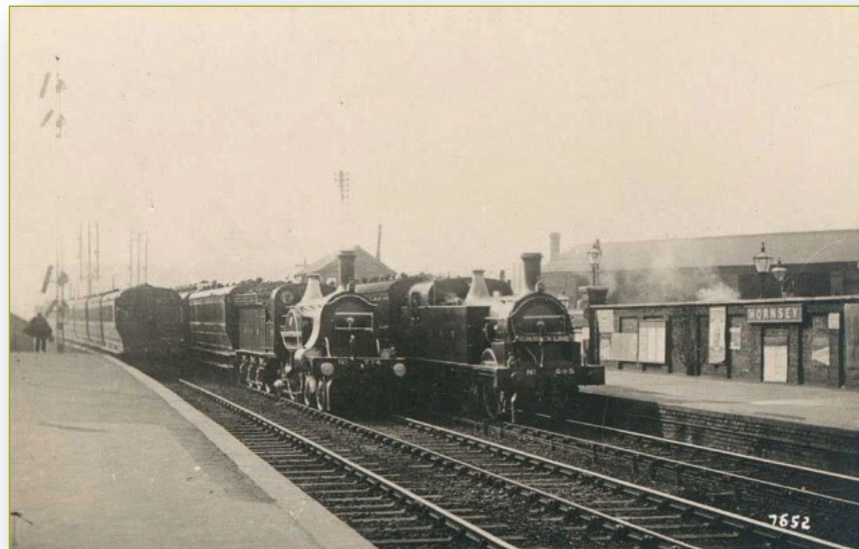
Hornsey Railway Station ▼
