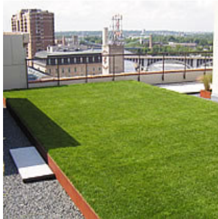
Figure 7 - Illustration of a Simple Intensive Green Roof
