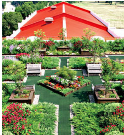
Figure 6 - Illustration of an Intensive Green Roof
