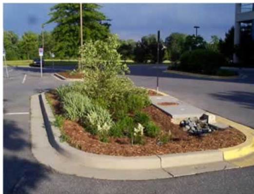
Figure 11 – Illustration of an engineered bio-retention area
