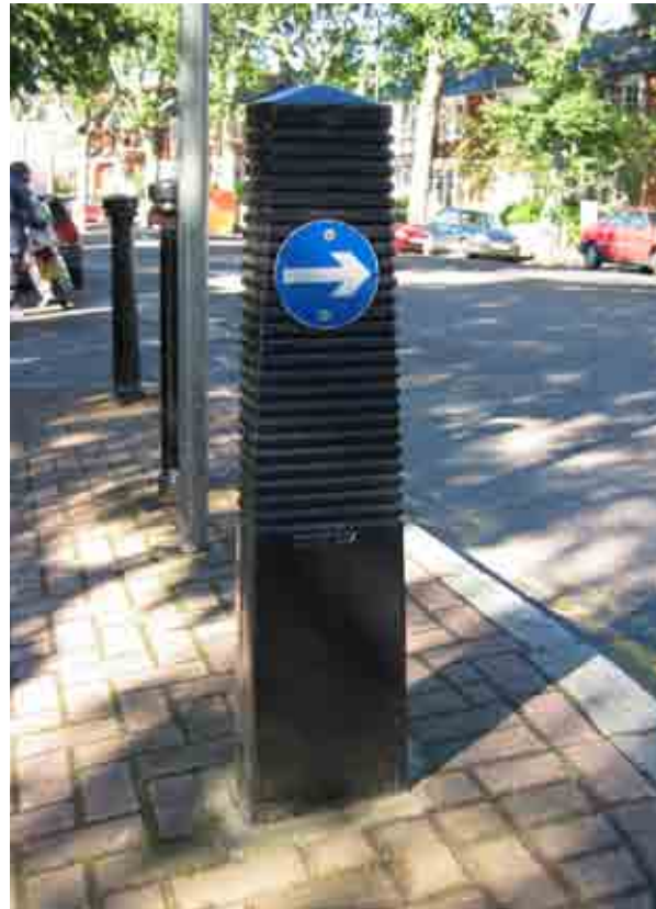
Consolidation of directional sign on bollard, Highgate
