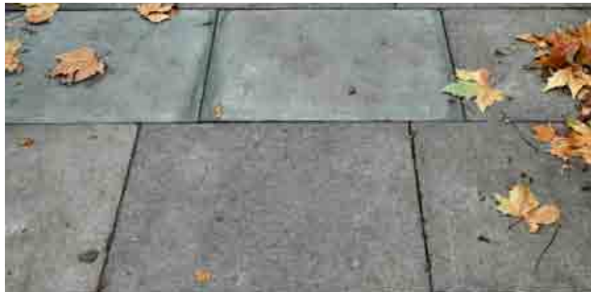
Use 600mm x 900mm concrete paving slabs along the High Road for consistency
