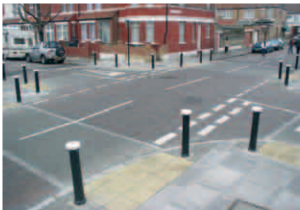
Junction treatment, Haringey
