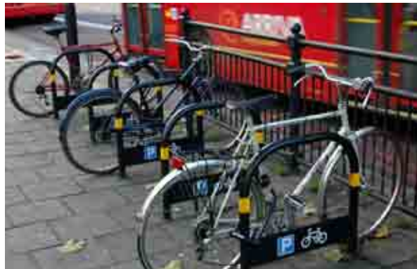
Sheffield Stand with crossbar with cycle parking signage
