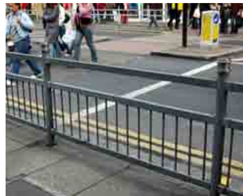
Wood Green Town Centre - Linx 200 3/4 height, post with stainless steel cap height
