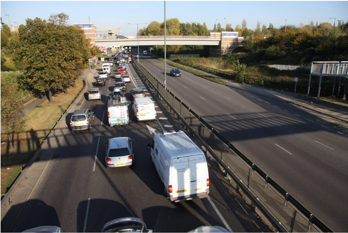
Figure 1: Tailback as Traffic Narrows from 3 to 2 Lanes on Approach to Bounds Green Junction. Note Pinkham Woods to Right of Picture
