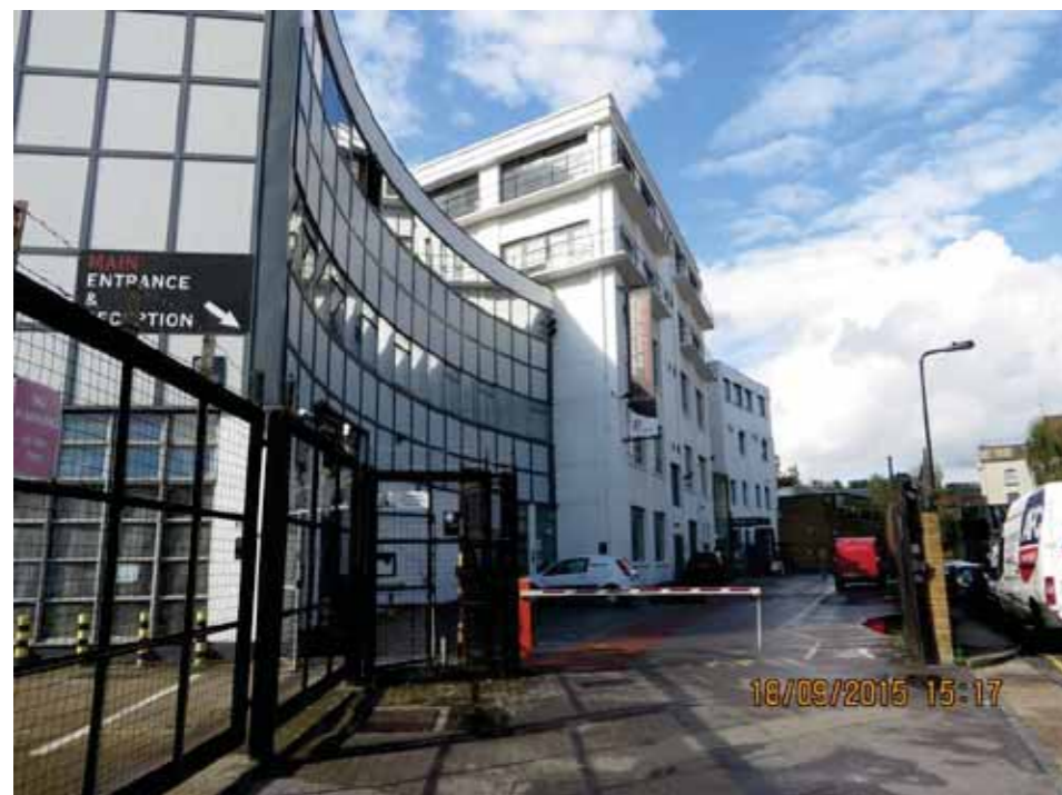
Figure 2: Chocolate Factory Car Park Access
