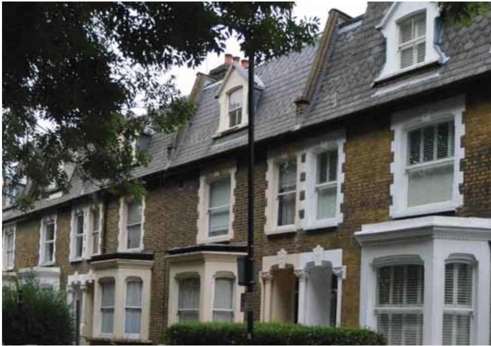
Terraced houses, Wood Green Common, Conservation area
