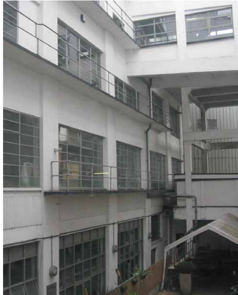
Internal courtyard, view looking west
