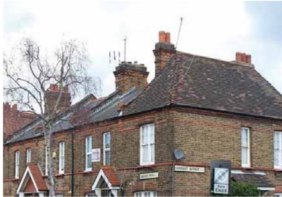
Terraced houses, Noel Park, Conservation area
