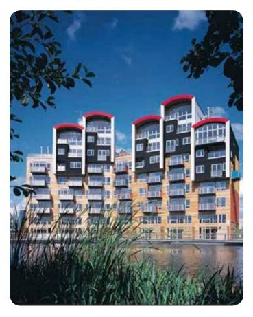
With large scale fabric improvements, additional insulation to metal stud wall constructions, roof and ground floors, high performance aluminium composite and timber windows the properties are far more energy efficient. This is a major factor towards the 44% increase in energy efficiency since 1999. Moreover building design allows maximum natural light combined with low energy lighting along with more natural ventilation.
