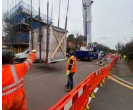
A crane lifting a bathroom pod
