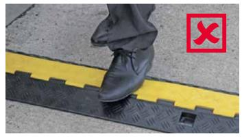
Figure 4. Cable protectors sit on top of the cable. This is still a health and safety hazard and is not permitted.
