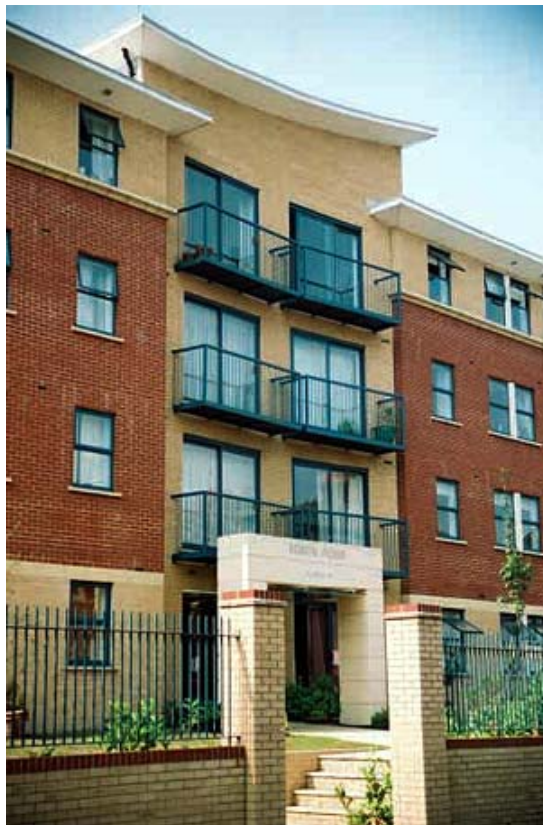
North Point, Tottenham Lane
