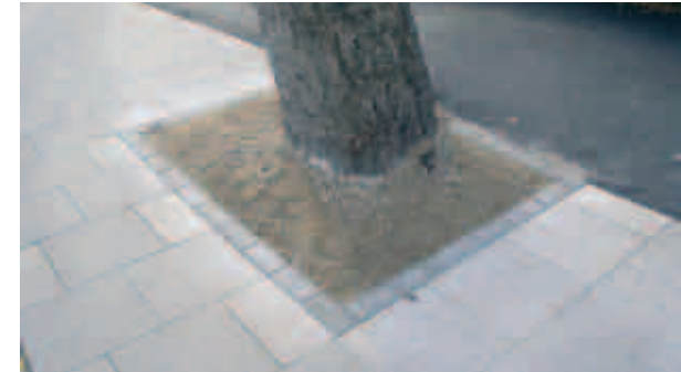
Good practice - porous resin bound gravel tree pit
