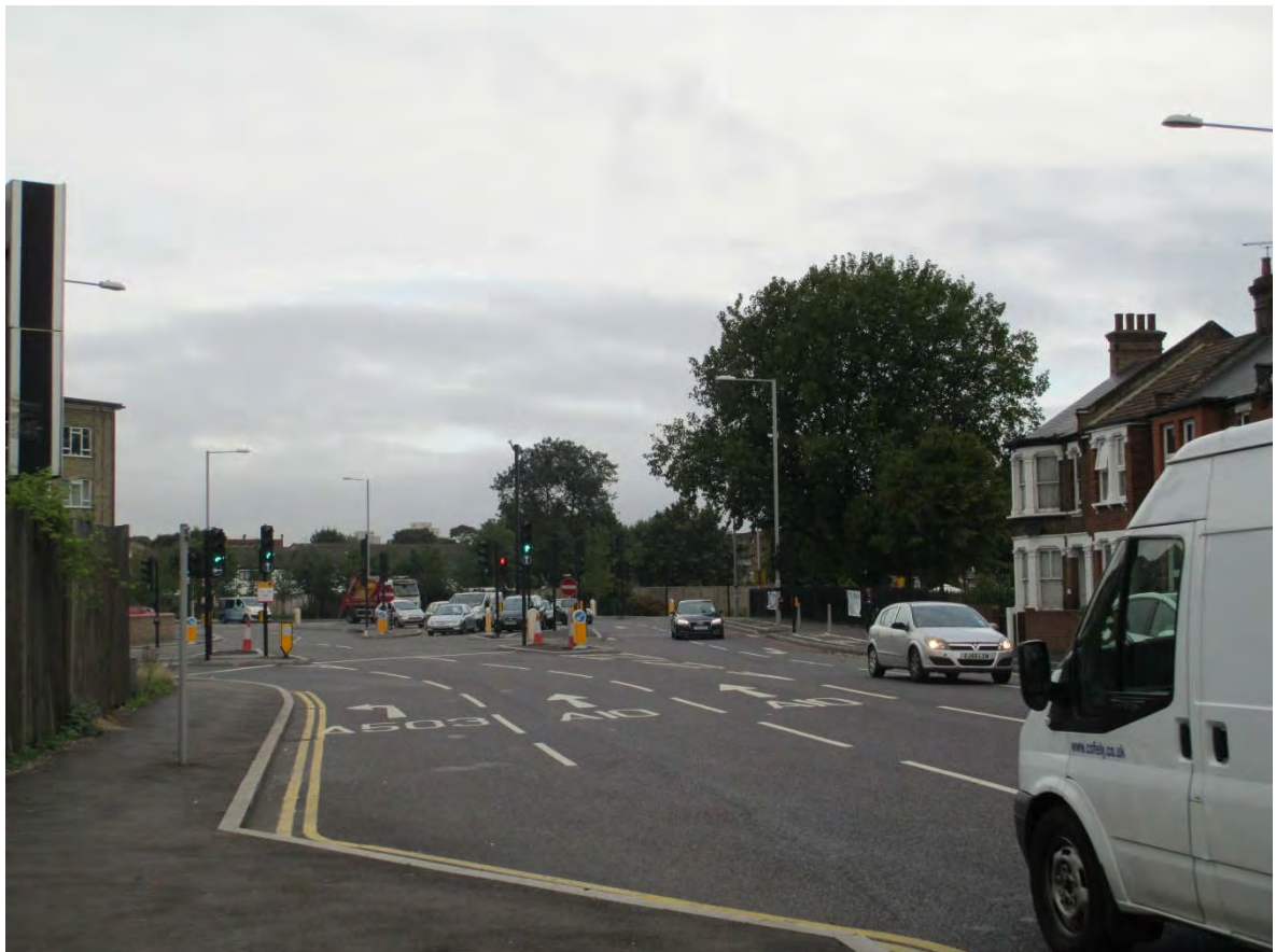
Figure 3.1: Junction of Watermead Way and Monument Way
