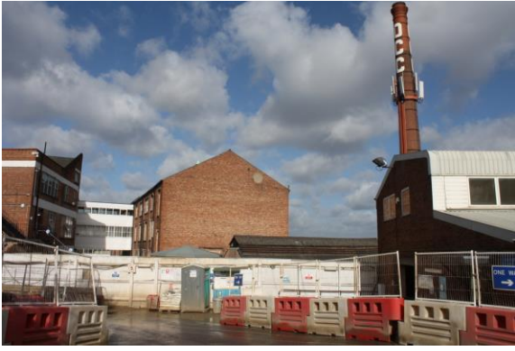
Eade Road grid work
