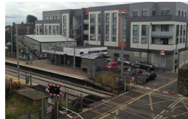
Station, level crossing and adjacent 4 storey residential
