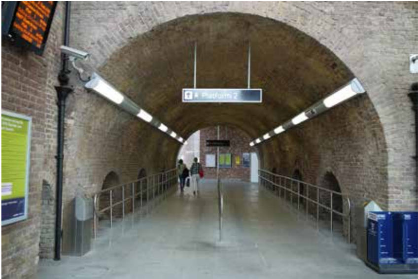
Unpaid pedestrian link beneath the viaduct
