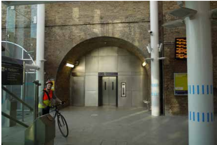
Arches used to house key station facilities
