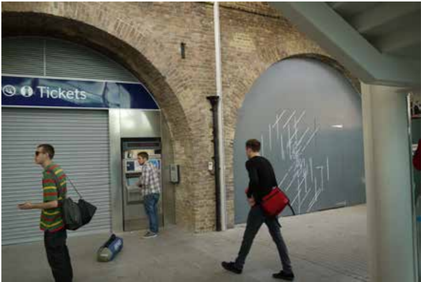
Arches used to house key station facilities
