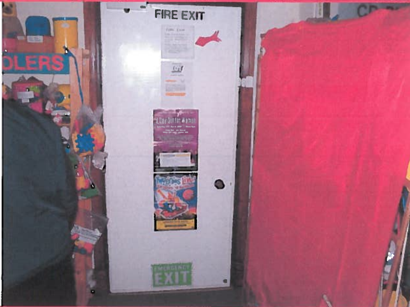
Panel lining to back of door
