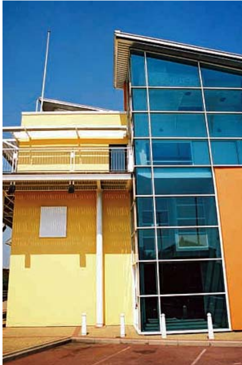
Heron House, Hale Wharf
