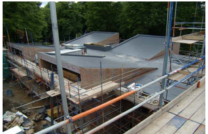
New sarnafil roof covering to the single storey building
