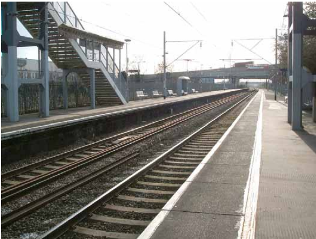
Figure 4.5 Angel Road Station
