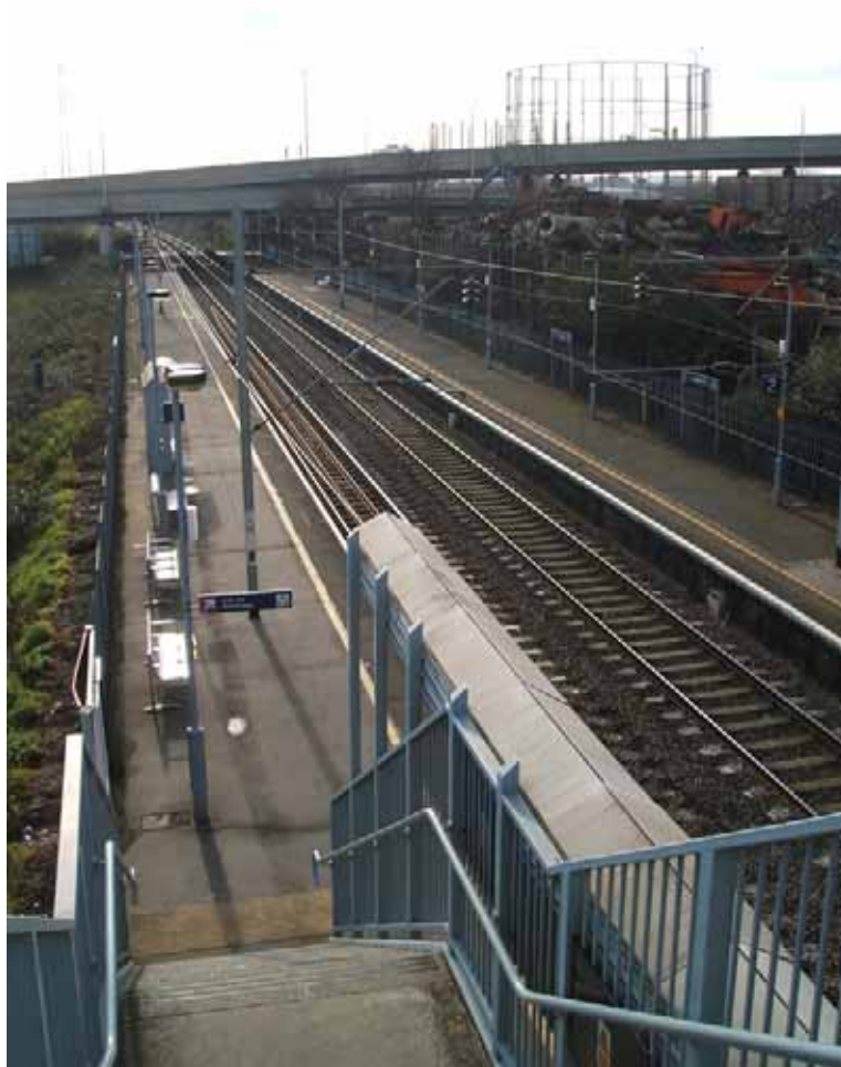
Figure 4.2 Angel Road Station
