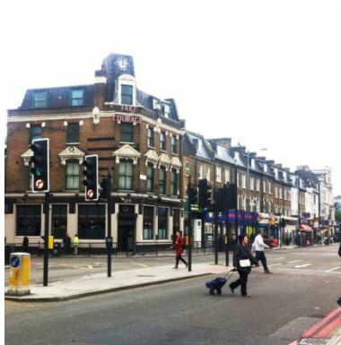
Photo 19: Intact historic block
