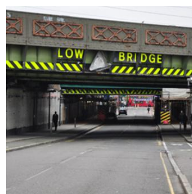
Photo 12: Bridge, Stroud Green Road
